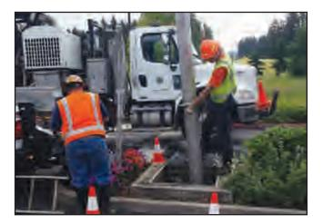
**4.** Using a small lift or the boom of the vacuum truck, remove the used cartridges by lifting them out.
