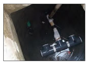
**9.** The used BayFilters must be sent back to BaySaver Technologies for exchange/ recycling and credit on undamaged units.
