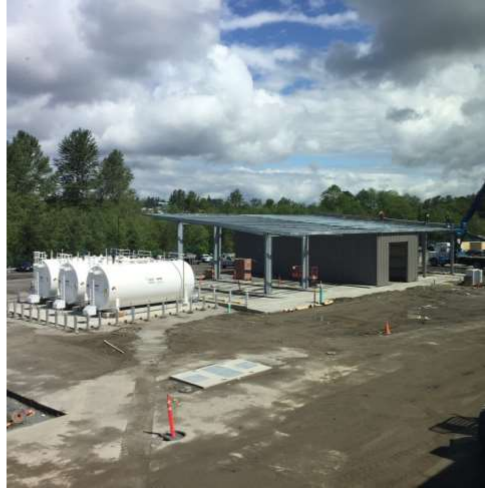
Fuel Island & Bus Wash
